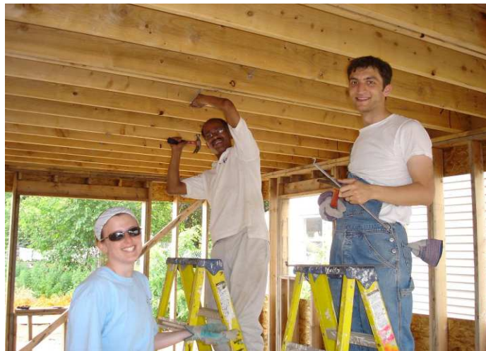
Members from a Hillier Architecture Team Build .
